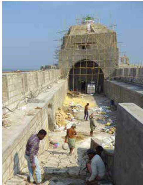
TOP TO BOTTOM: Relaying of stone floor at Pani Kotha; Cut outs acting as skylights in the Naida Caves; View of the Audrey House (after restoration).
